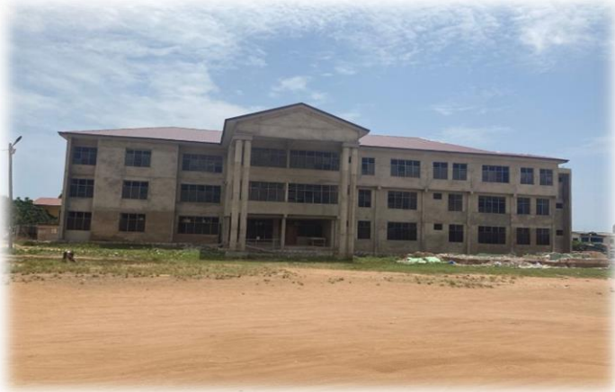
CONSTRUCTION OF OFFICE BUILDING COMPLEX (80% COMPLETED)
